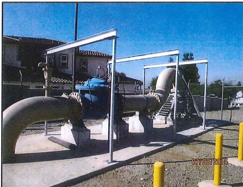
Progress photo to show the installation of the structural steel members
