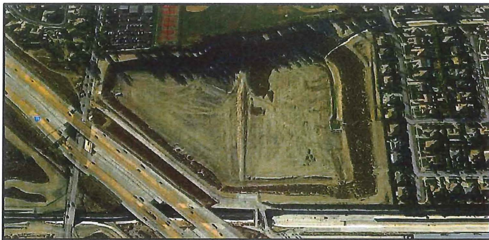
Aerial of Victoria Basin
